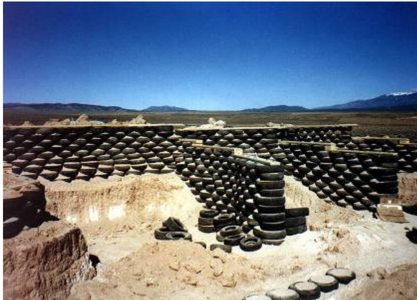
Figure 3: Nest modules under construction in Taos, New Mexico (Earthship Biotechnology cited in Howarth, 2004).
