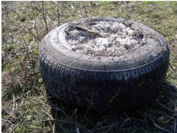
Figure 5 (left): Unit of construction, a tyre rammed with local chalk from the Brighton Earthship (Howarth, D 2004).
